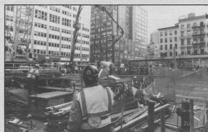
Construction of Four Seasons Hotel New York Downtown.
